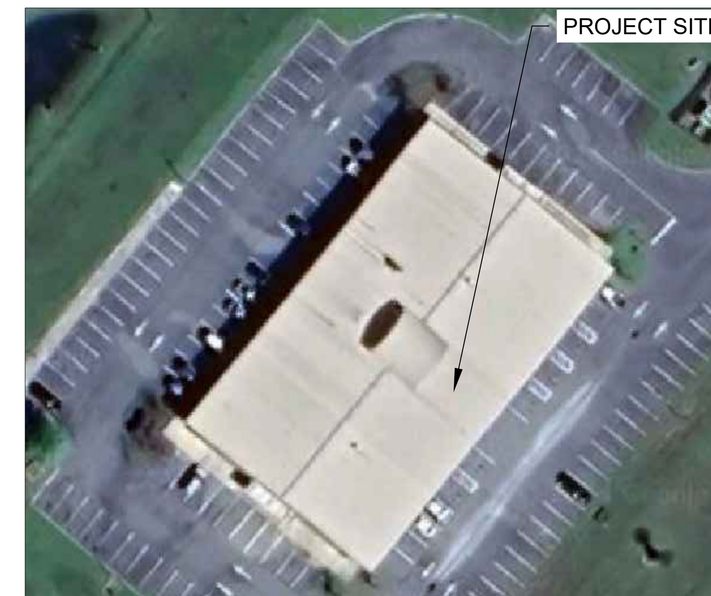
1 BUILDING PHOTO SCALE: NTS
